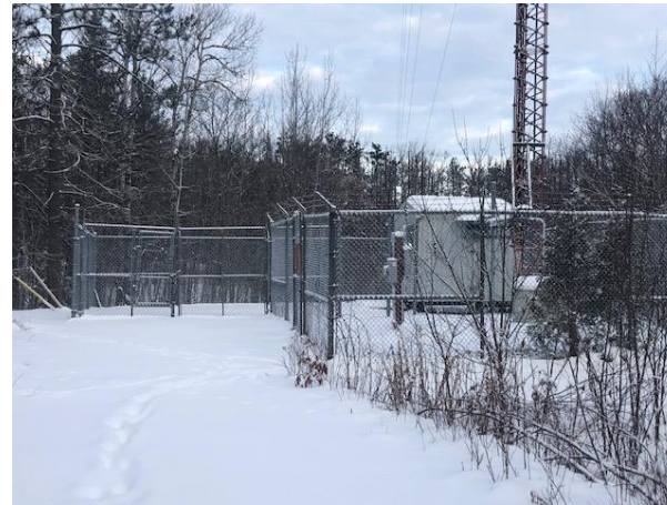
The radio base station equipment, UPS, and other supporting equipment was also upgraded as part of this project.
