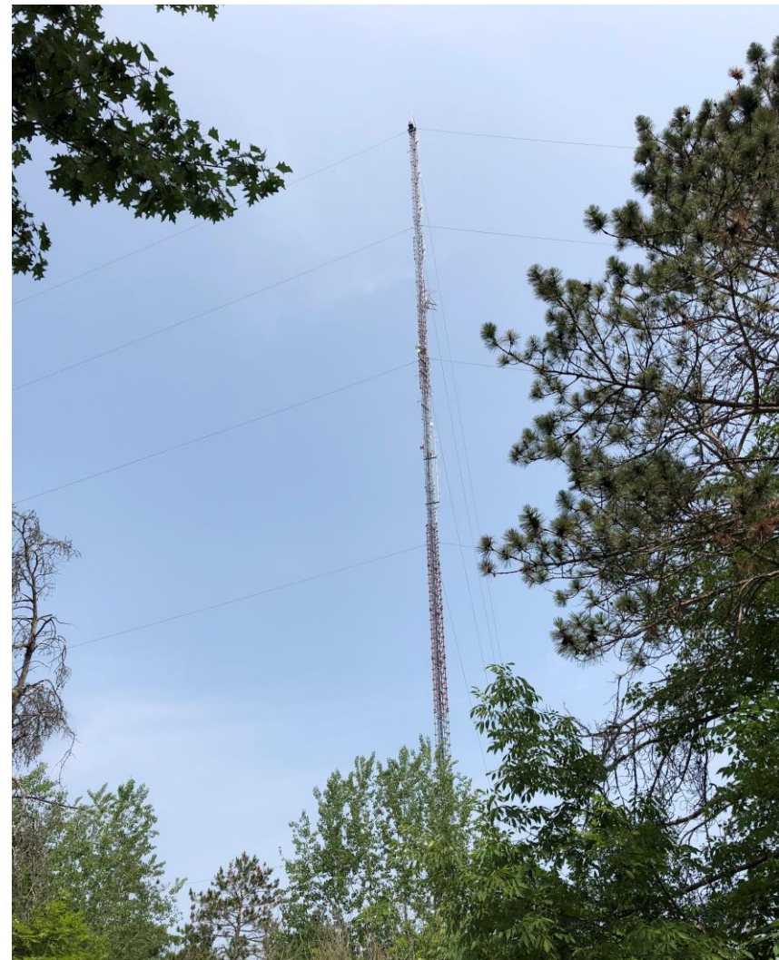
Upgraded existing 200 ' SMART Tower
