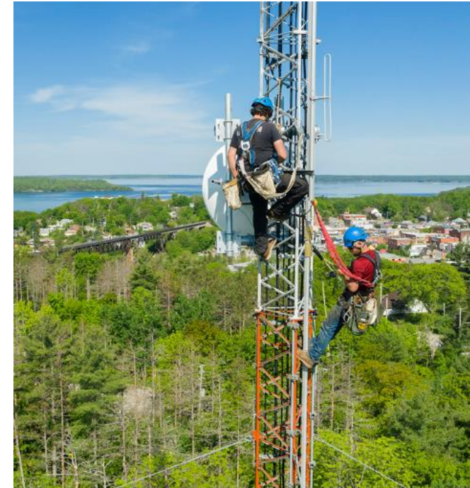
Old radio equipment was removed as part of the project, replaced with 15Gbps microwave radios to connect to the new Carling Township tower 13 km away.
